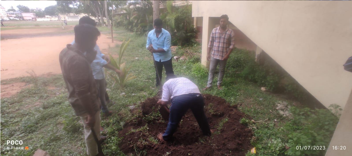
RAIN WATER HARVESTING 11-06-2023
